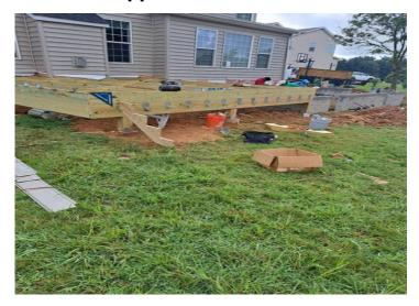
**Construction Step 4**Step 4: Building the frame of the new addition.
